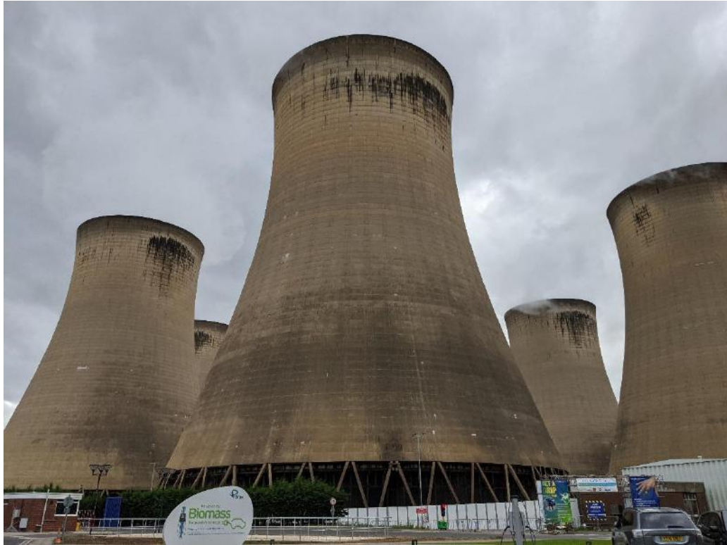
Photo 1: Cooling towers located in the northern section of the Drax Power Station site. Photo taken looking towards the north.
